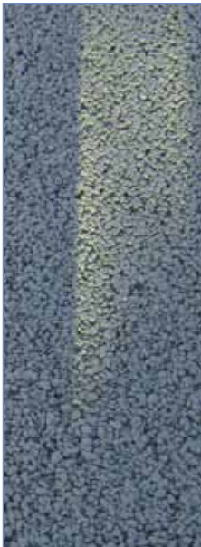
To reduce stormwater runoff, use permeable material, such as the pervious concrete shown, to construct trails, sidewalks, parking aisles or other paved areas.
